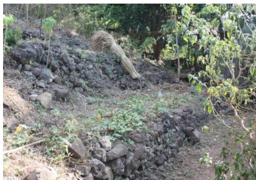
Figure 2. Terrace Structure in Homegardens
