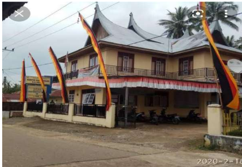
Gambar 4.1 Kantor Wali Nagari Balimbing
